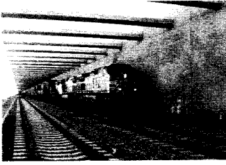
THE MID-CORRIDOR TRENCH. PHOTO COURTESY ALAMEDA CORRIDOR TRANSPORTATION AUTHORITY.
